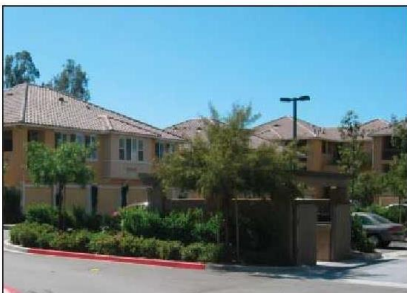
3.2.5.7 a) Trash enclosures with landscape screens and architecture that is similar to that of the project help to minimize the negative visual impact of these structures.
