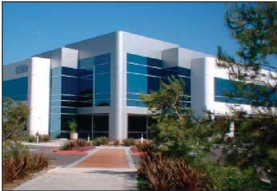
3.3.4.4 b) Quality building materials enhance the look of office/business parks.
