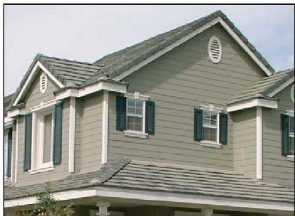
3.3.7.1 b) Facade articulation such as the use of dormer windows add richness to both the home and the streetscape.
