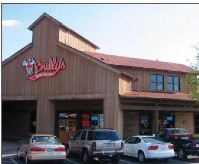
3.3.3.5 a) Natural looking materials such as wood add authenticity to buildings .
