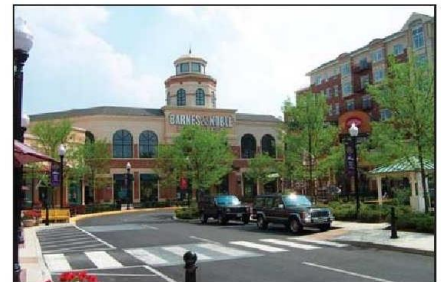
3.2.3.1 e) Icon buildings located at prominent locations will help build an identity for the village center.
