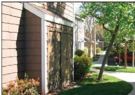
3.2.5.7 d) The screening of utilities can be integrated into the adjacent building through the use of similar materials and architectural elements.
