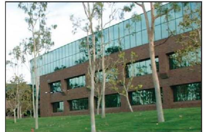
3.3.4.1 g) Variations in façade color and material increase the attractiveness and quality of business park development.
