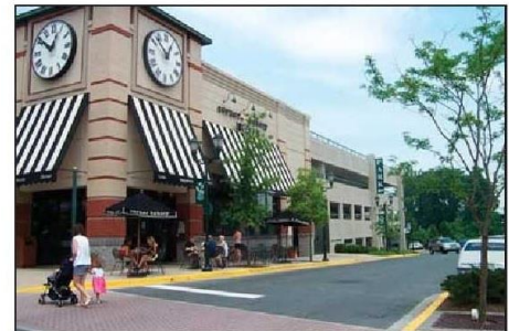
3.2.3.4 f) Parking structures on side streets, directly behind retail uses, provide convenient access and preserve pedestrian street environment.
